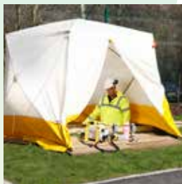
Welding tent/shelter and ground sheet
