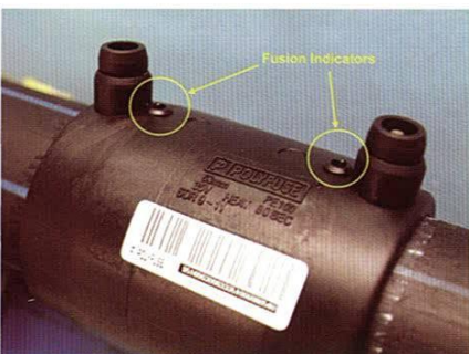
[ 11 ] Ensure fusion indicators are raised. This indicates successful completion of fusion process.
