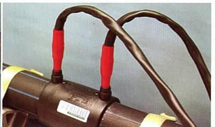
[ 9 ] Connect the welding cables to the fitting terminals.
